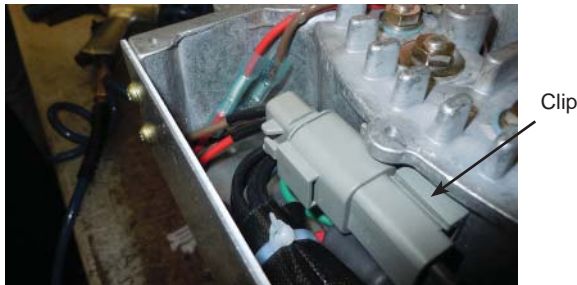
Figure 1 — Gray Field Connector Attached to Housing with Clip
